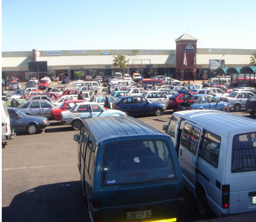
Kuyasa Mall and Taxi Rank at Mdantsane CBD. There are plans to extend the mall to increase the quality and quantity of the retail offering in the CBD, and include other uses in support of retail.
