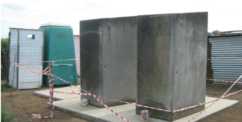
Chemical toilets replaced with waterborne toilets at Lillian Ngoyi informal settlement, N U 8, implemented by the Water and Sanitation division within Engineering Department.
